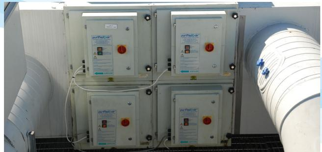
4 ESP Units Stacked in modular formation with a double pass
