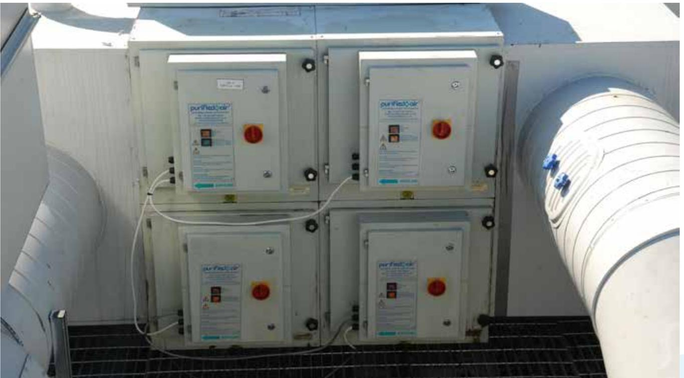
4 ESP Units Stacked in modular formation with a double pass
