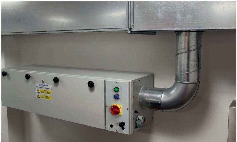
*Figure 6 - UV-O 1000 Unit Installed*
