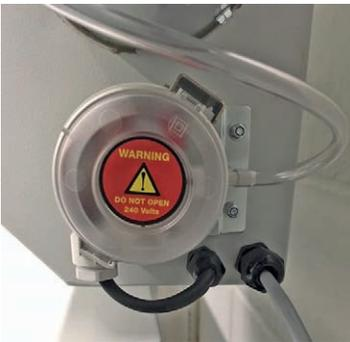
Figure 8 - Air Flow Sensor
