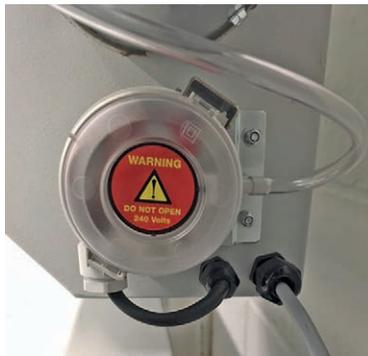
**Figure 17 - Air Flow Sensor**
